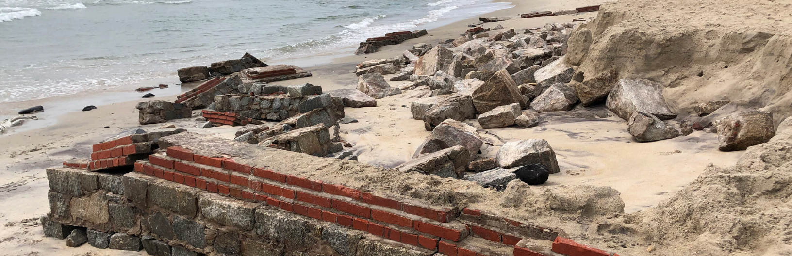
Original Cape Hatteras Lighthouse Fence Foundation Cape Hatteras National Seashore Photo
